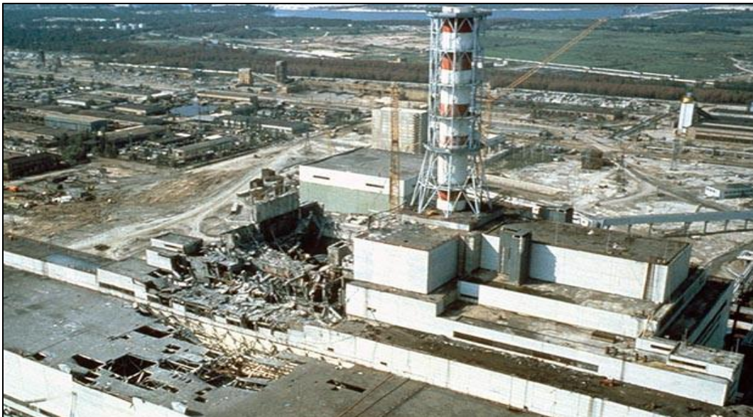
Fig. no.4.2-Reactor 4 site in weeks following the explosion, with damaged structures and fallout signs
